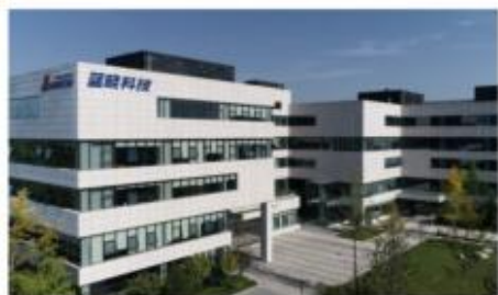
Sunresin Park, Headquarter
